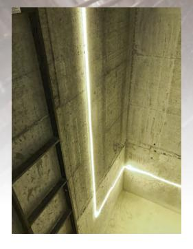
Equipped with prewired automatic switches. Light intensity complies EN81-20 requirements. Installation with dowels and clamp is faster than install traditional lighting installation.
