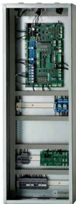
Logic and security control panel positioned in the shaft
